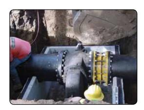
The DJ405's design eliminates restraint tie-rods with Romac's UL rated, FM approved RomaGrip™ to lock the spool piece into the desired position.
